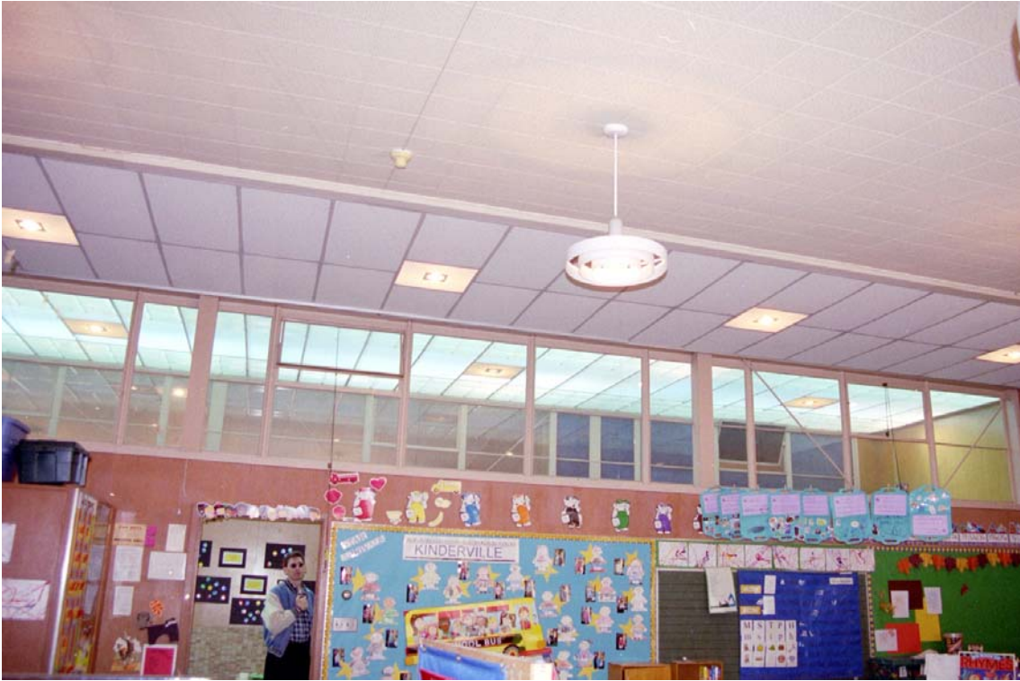
Figure 5: High Windows at Central Corridor with a Partial View of Diagonal Tie-Rod Bracing
