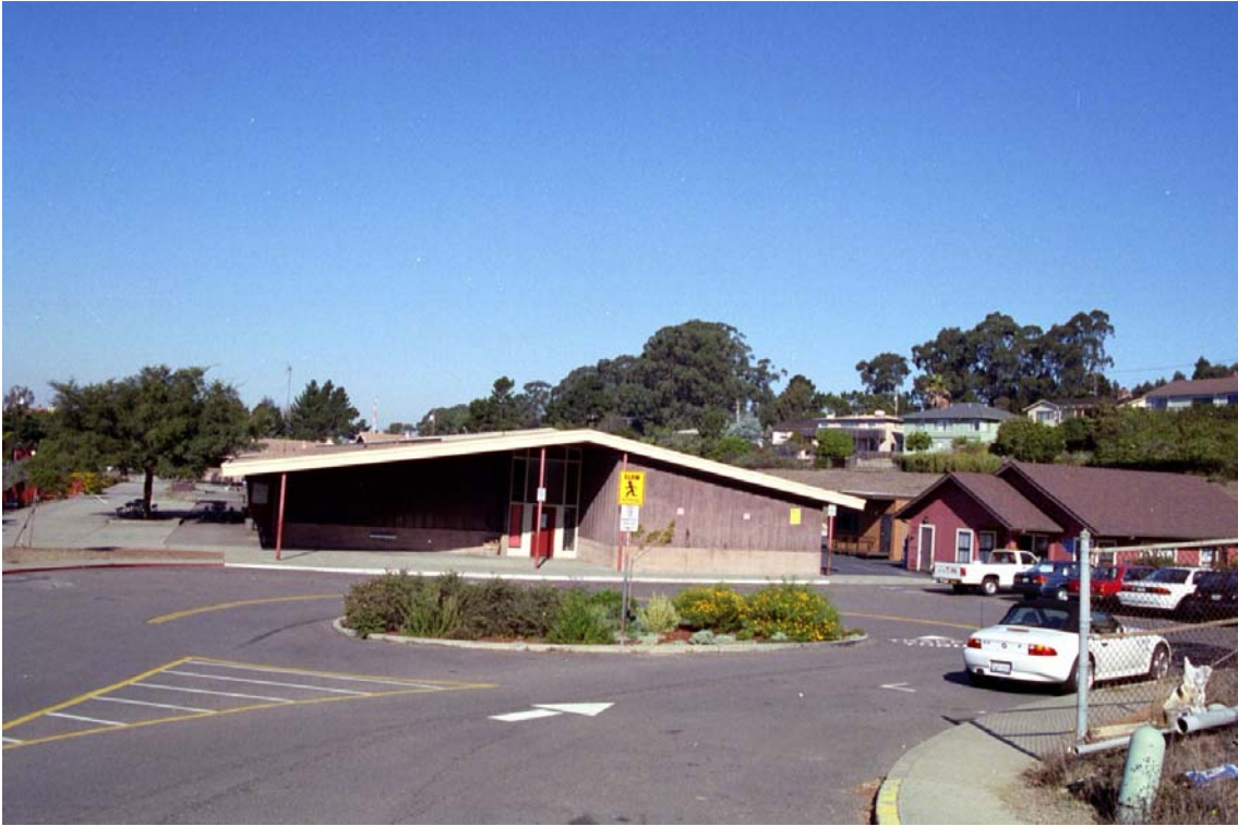
Figure 3: East End of Classroom Wing
