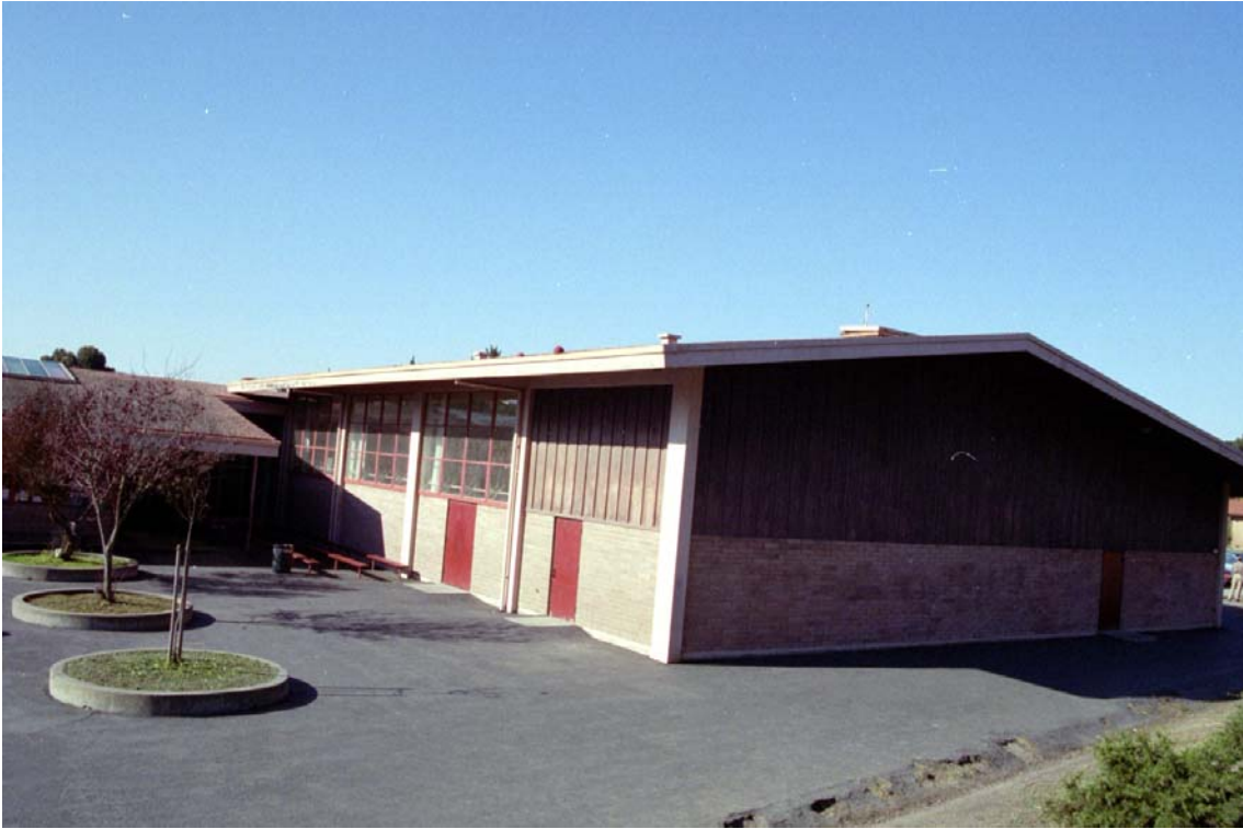
Figure 8: Northeast Corner of Multi-Purpose Room
