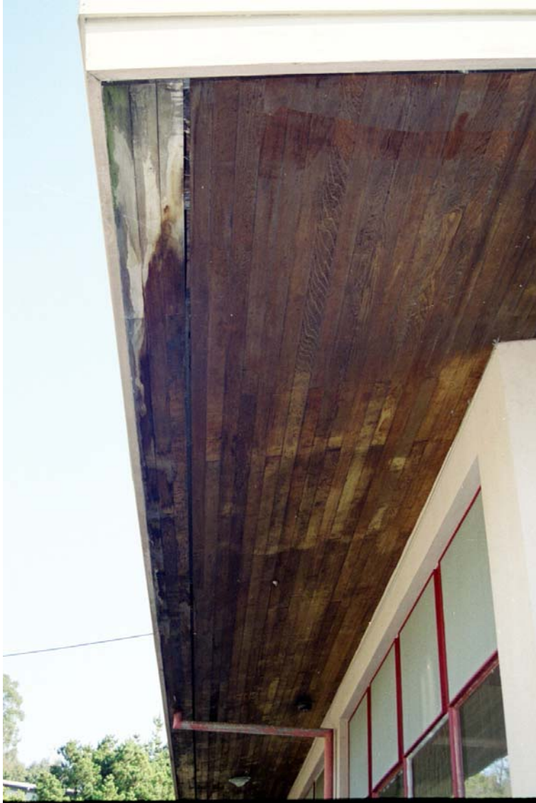
Figure 14: Deterioration of Wood at Soffit
