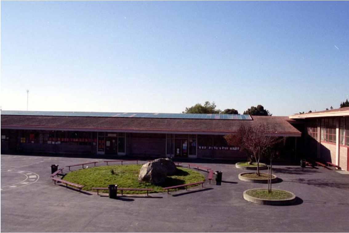
Figure 4: North Side of Classroom Wing
