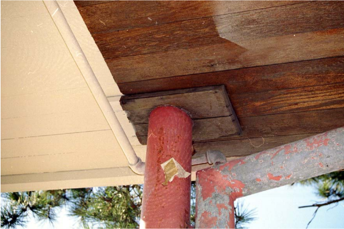
Figure 13: Rust at Exterior Pipe Column
