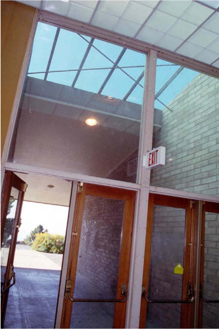
Figure 7: Tie Rod Bracing at Skylight Opening
